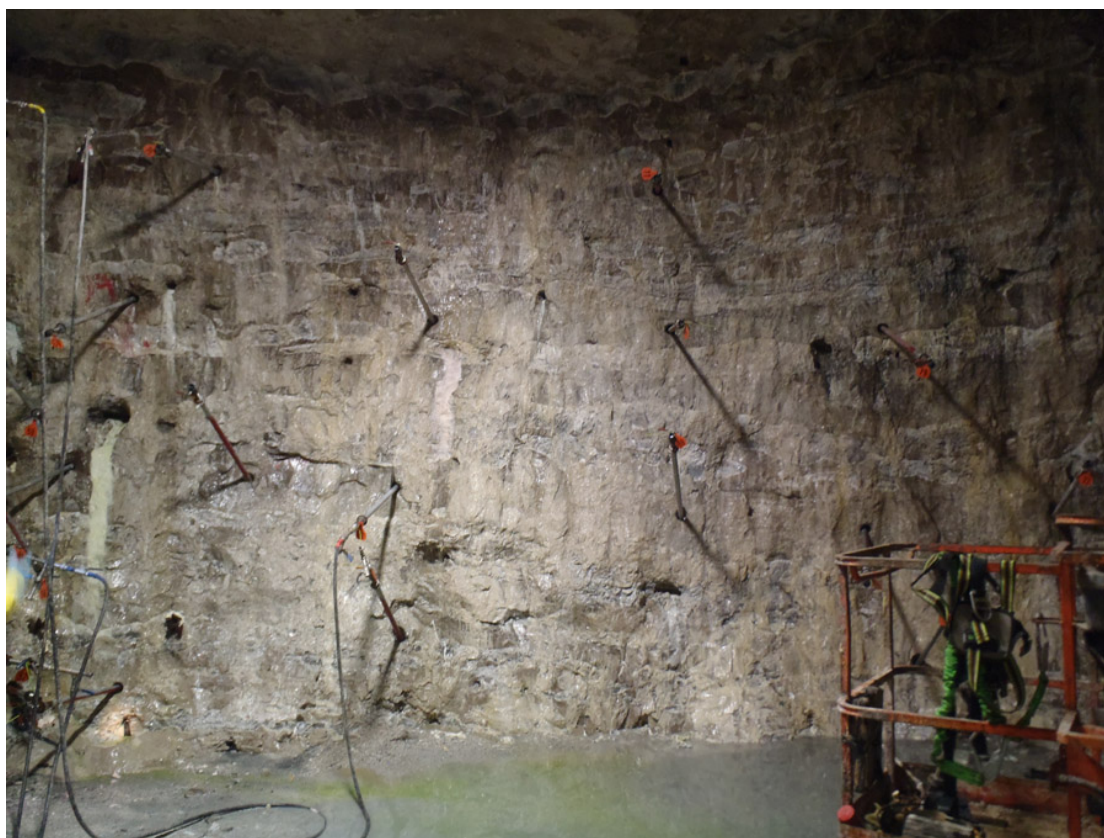
Figure 6. Randolph Mine grout face on belt slope
